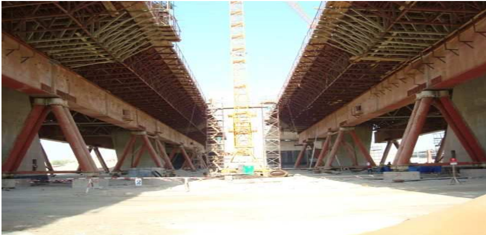
Fig.3 Construction of the deck using box girders and pipes
