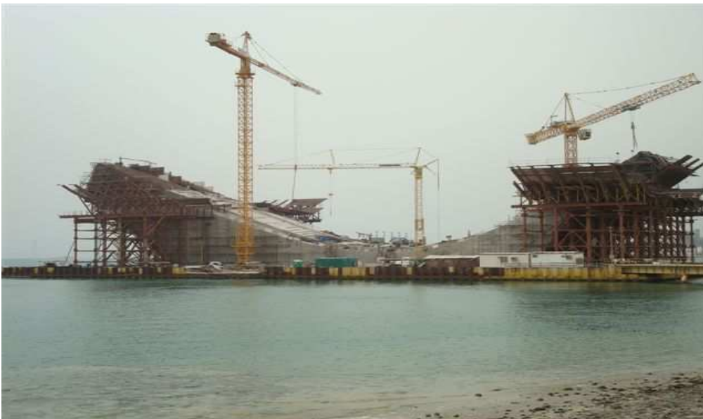
Fig.2 Construction of the central pier
