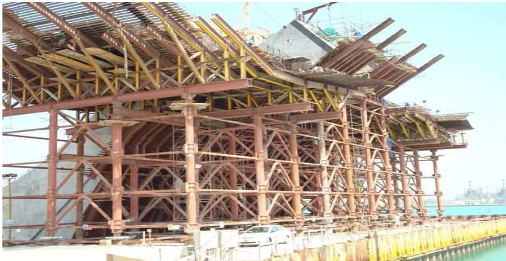
Fig.4 Falsework system for the construction of the piers
