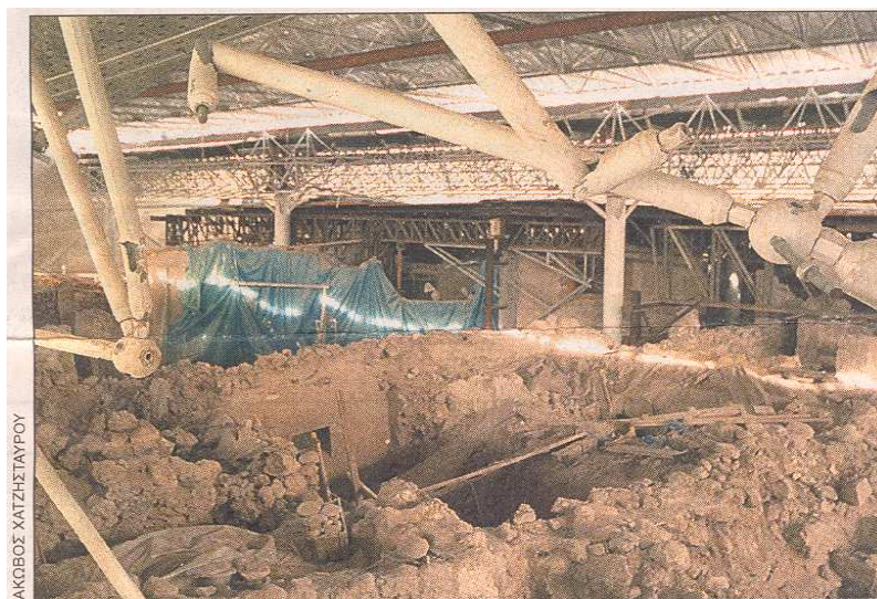
Fig. 2: Partial collapse of a steel space frame canopy, Santorini, 2005
