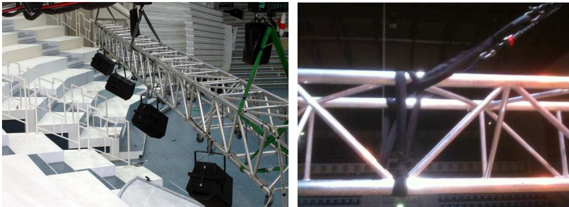
Fig. 1: The beams are often lifted by using polyester slings
