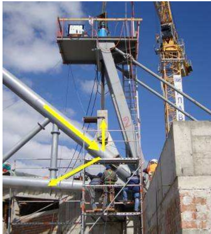
Fig. 31 Fixing of the main supports
