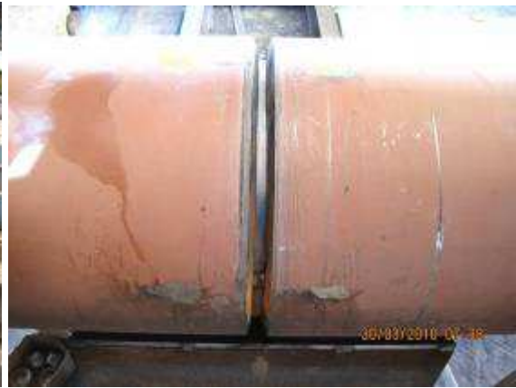
Fig. 17 Butt welding preparation
