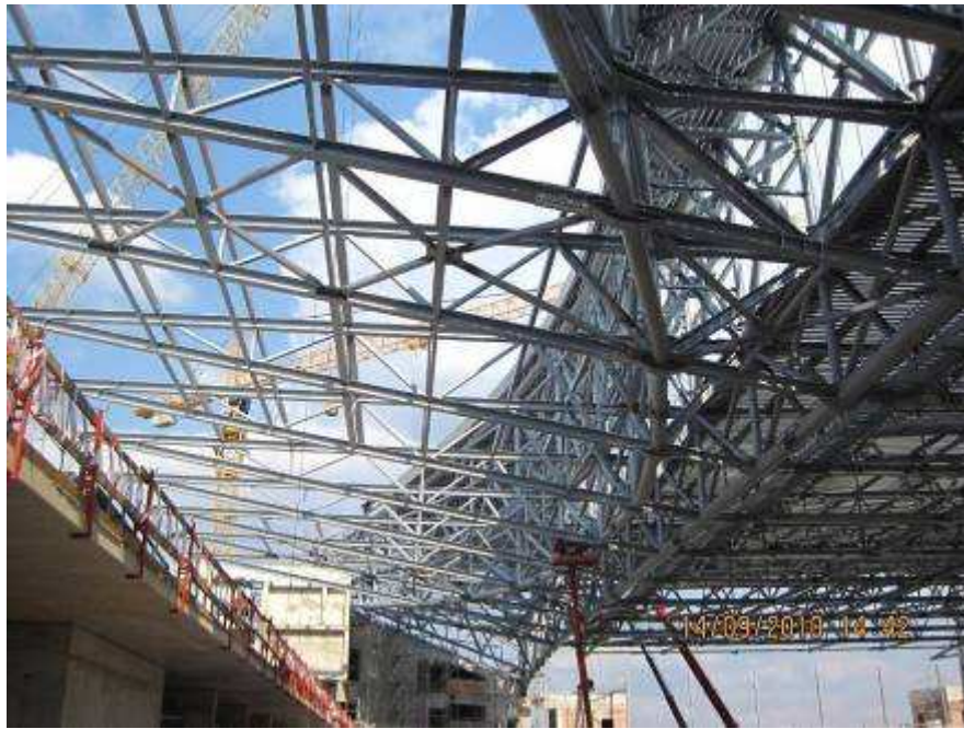
Fig. 36 Erection of the triangular trusses
