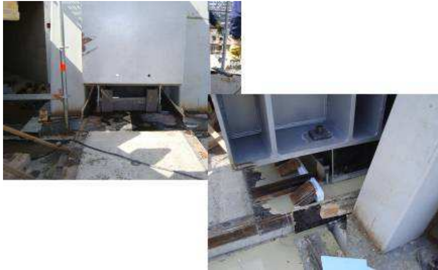
Fig. 33 Fixing of the bearings
