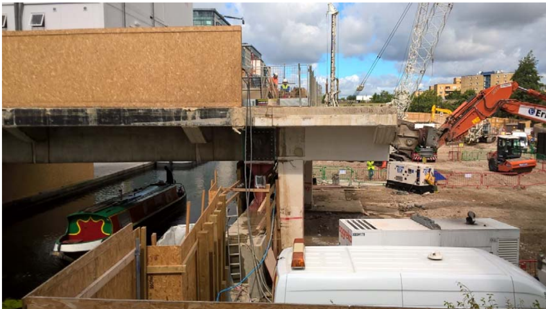
Fig. 8 Wire Cutting part of bridge to be demolished while boat crosses
