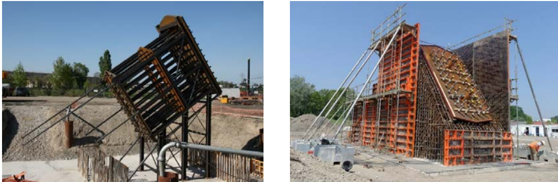
Fig. 10 Support of the arch anchorage © EIFFAGE METAL
