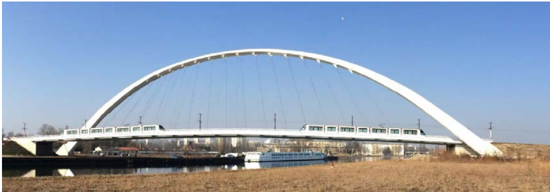
Fig. 2 South view of the Citadelle Bridge © EGIS
