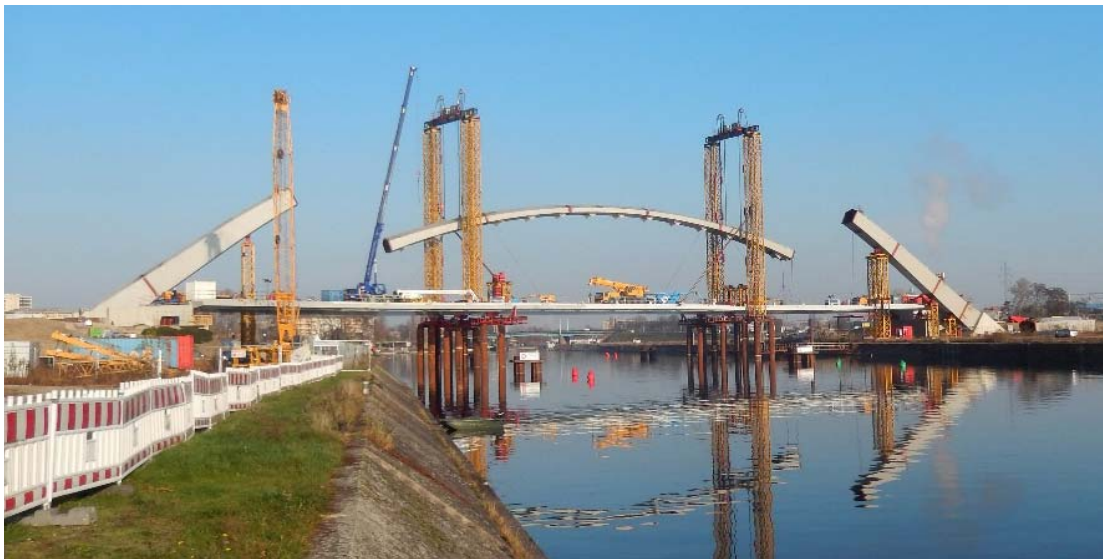
Fig. 12 Lifting the central part of the arch © EIFFAGE METAL
